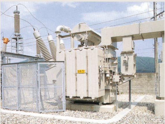
Oil-immersed transformer
