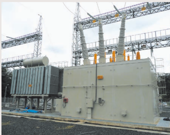
Roof-delta connection transformer
