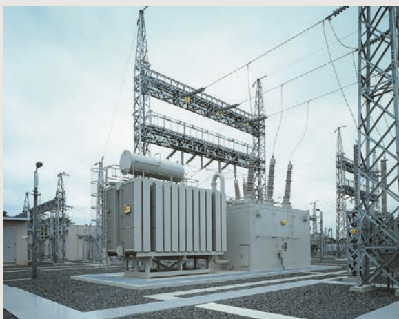
154 kV Scott connection transformer
