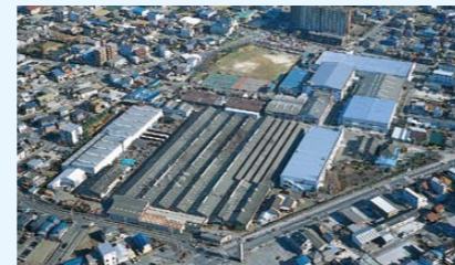
Meiden Nagoya Works
