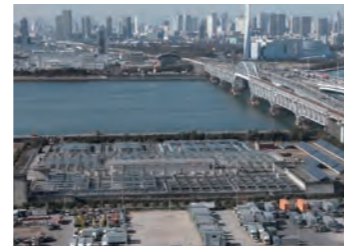
Overall facility view on south side
