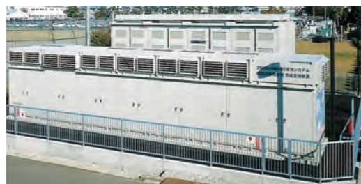
PCS for NAS batteries
