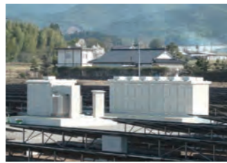
Power conditioner (right) and high-voltage joint facility (left)
