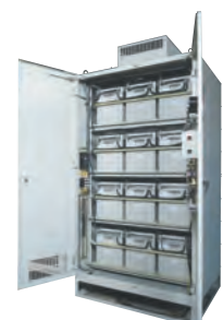
Regenerative power storage system (CAPAPOST)
