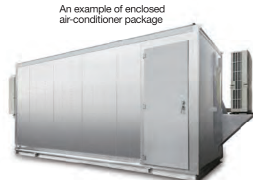
Applicable conditions: Minimum temperature of a year -15^{\circ}\text{C} (optional) Coastal area where salt damage is anticipated
