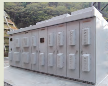
1MW SVC (delivered in 2012) ▶
