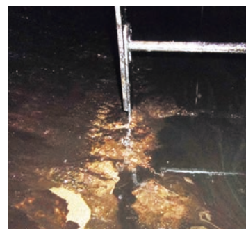
Contamination in the fuel tank
