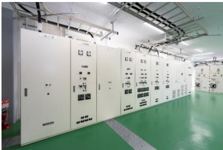
Monitoring and Diagnostic System for Power Receiving
