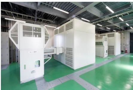
Silicon Rectifier and transformer for the rectifier
