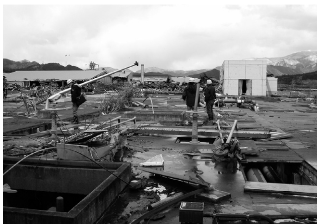
Fig. 3 Situation of Damage at the Upper Area of the Site in the Ofunato WPC
