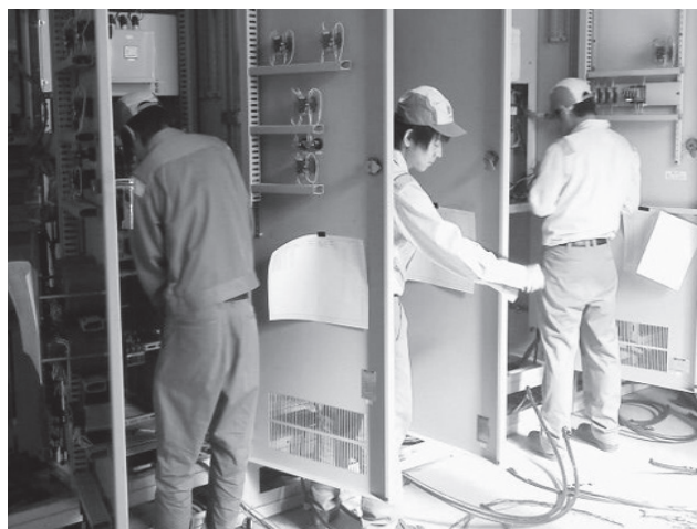
(a) Training for cable connections
