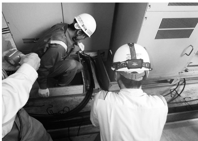
Fig. 7 Training for Cable Removal Work
