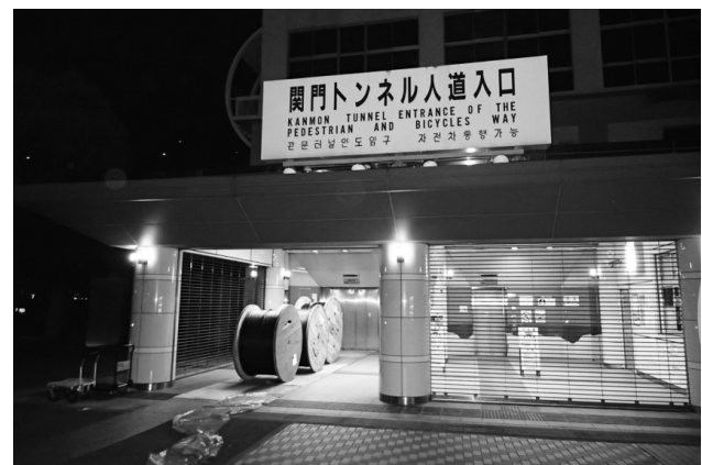
Fig. 4 Cable Drum Carry-in for Cable Laying in the Tunnel
