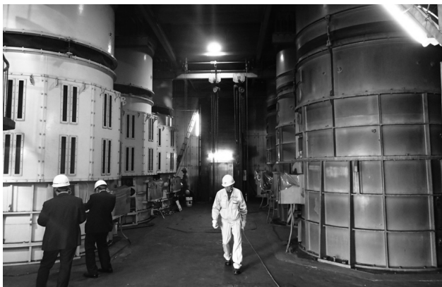
Fig. 2 Ventilation Facility before Replacement at the Kojo-Side Shaft
