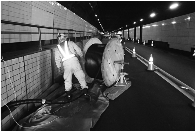
Fig. 5 Cable Laying Work at the Pithead of the Tunnel
