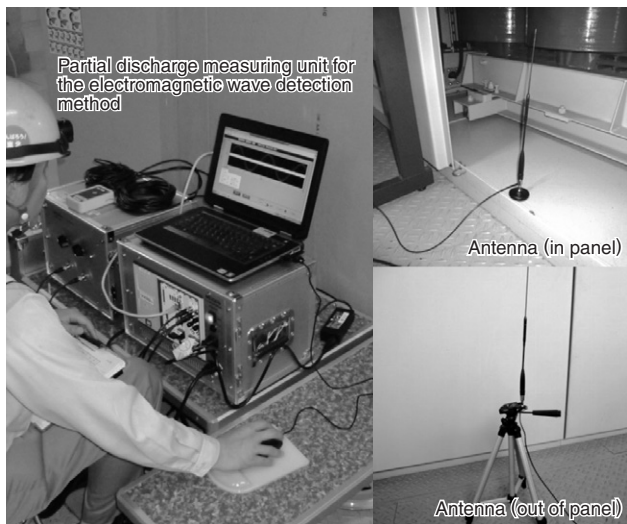
Fig. 7 View of Partial Discharge Measurement by Electromagnetic Wave Detection
