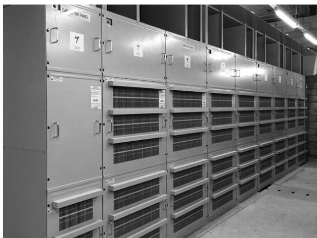
Fig. 3 Capacitor Panel
