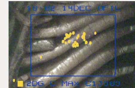
Rotary machine stator coils
