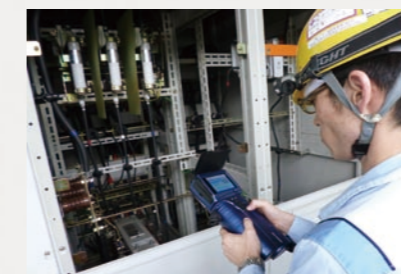
Examples of diagnosis using a corona camera
