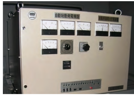
New panel after renovating
