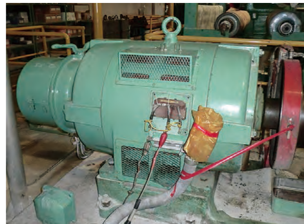
Insulation diagnostic test
