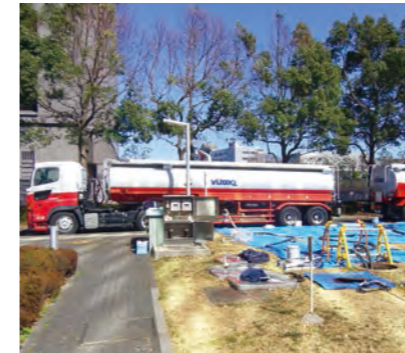
Inspection of a 100KL underground fuel tank
