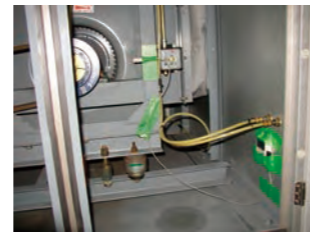
Temperature and humidity telemetry (for a fixed period)
