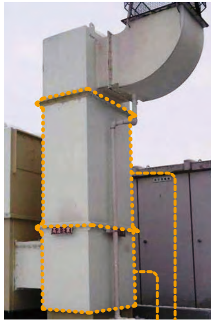
Inspection of an exhaust duct
