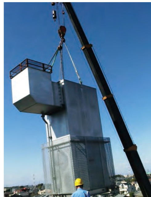
Renovation of an exhaust duct
