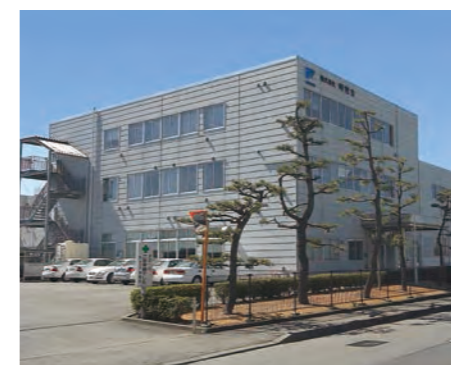
Meiden Engineering Center
