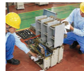
Inspection of vacuum circuit breaker
