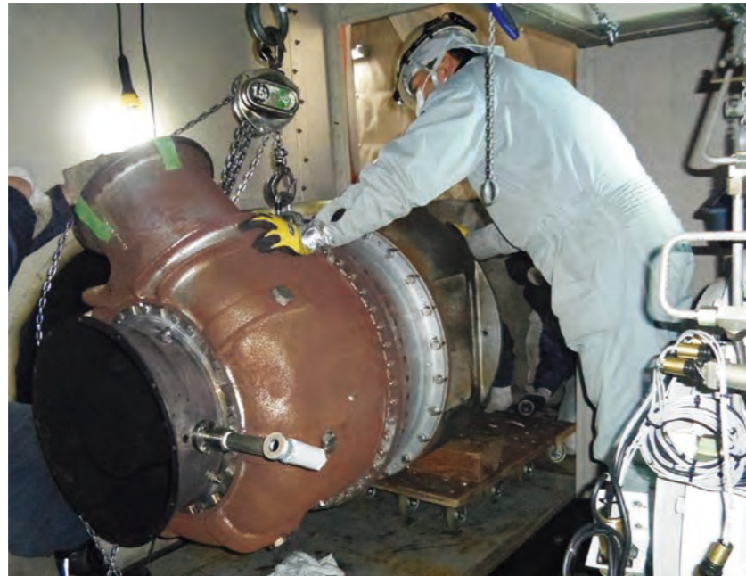
Gas turbine being overhauled
