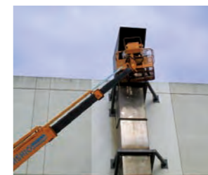
Regular inspection for the gas-turbine exhaust port
