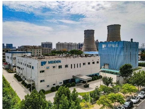
Photo right: Exterior of the factory of Meiden Zhengzhou Electric Co., Ltd.
