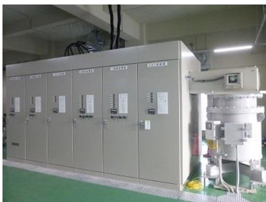
Gas-insulated switchgears
