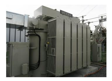
The product, which uses plant-based palm fatty acid ester (palm oil) for insulation, can be transported fully assembled and fully loaded with palm oil. The company also plans to deliver transformers using natural ester oils, such as soybean oil and rapeseed oil, for which TEPCO PG has placed orders, in addition to those filled with palm oil.
