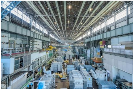
Overall view of the transformer factory
