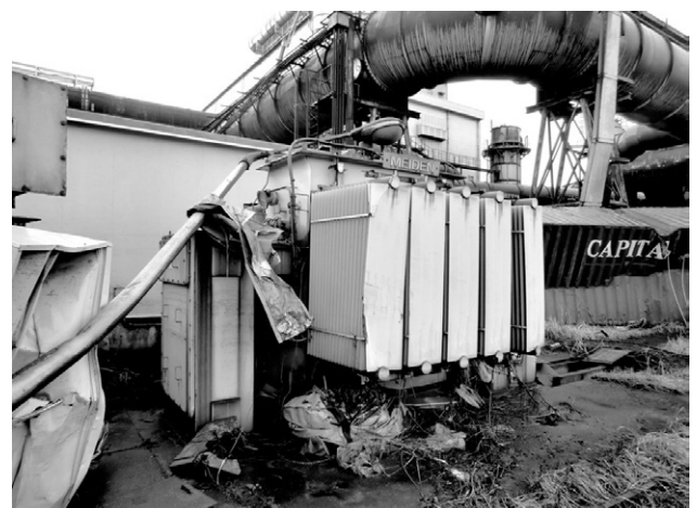
Fig. 6 Destroyed Transformer
