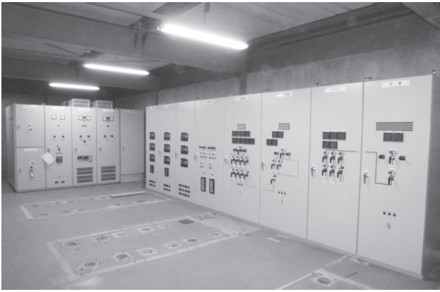
Fig. 8 Restored Field Monitoring Panel
