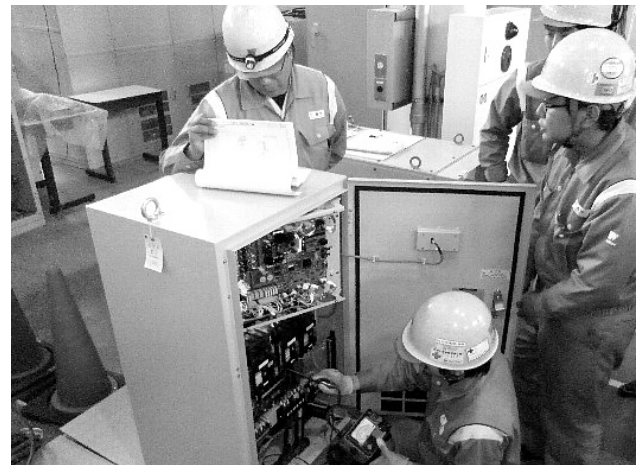
Fig. 7 Training for Power Conversion Equipment
