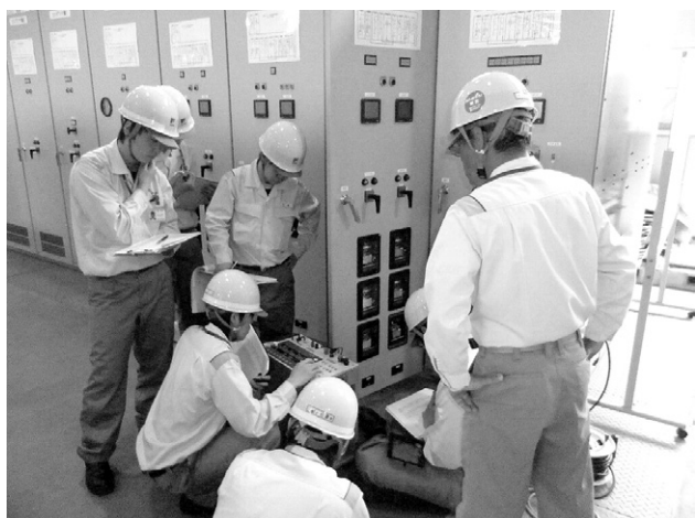
Fig. 2 Training for Protection Relays
