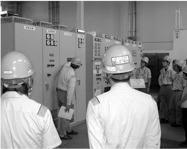
Fig. 12 Training for Power Conversion System
