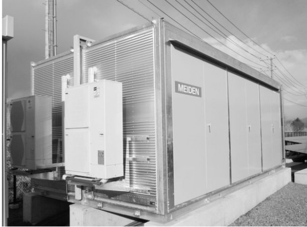
Fig. 2 PV Inverters
