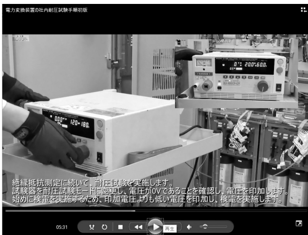
Fig. 6 Example of Working Procedure Explanation by Withstand Voltage Test Video
