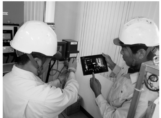
Fig. 9 Inspection Patrol Scene and Inspecting Members Refer to Inspection Method Video
