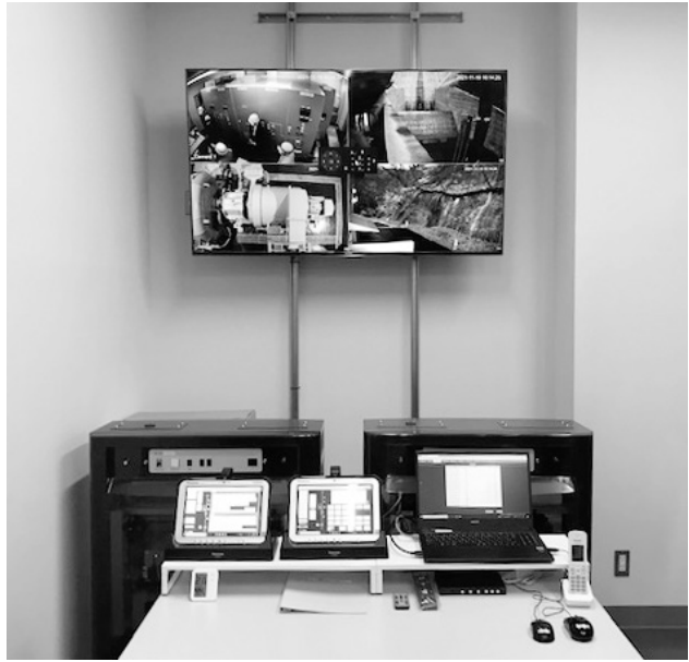
Fig. 4 Next-Generation Control Panel and Large Display
