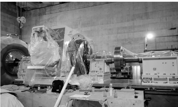
Fig. 9 Insertion of Rotor
